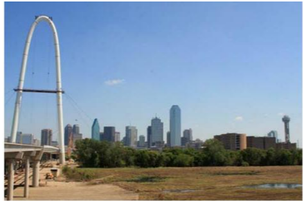
MARGARET HUNT HILL BRIDGE CONSTRUCTION, SEPTEMBER, 2010
