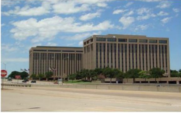
Western Place, Fort Worth
