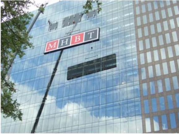
MHBT signage going into place, June 2010
